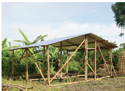
Structural skeleton of a house, showing cross-bracing
